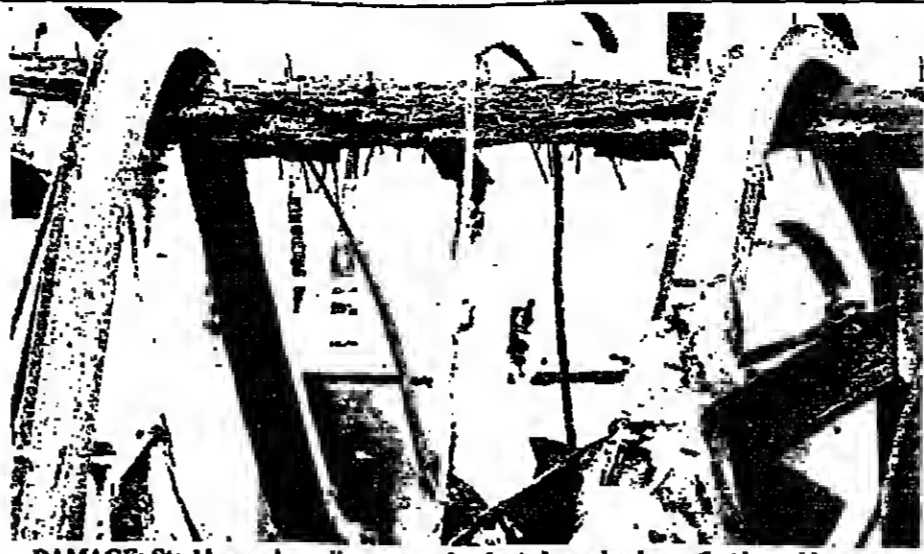
DAMAGE: Steel beams hang limp over a laminated wooden beam that has withstood a devastating fire. Danish officials are working to present a seminar to discuss fire safety with local agencies.
